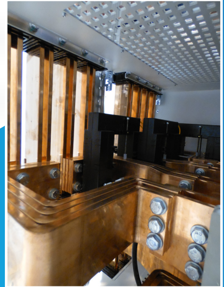
Example of a new modular switchboard
